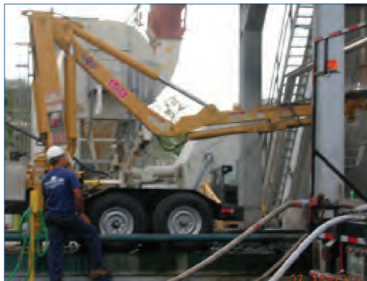
ASPHALT SILO CLEANING
