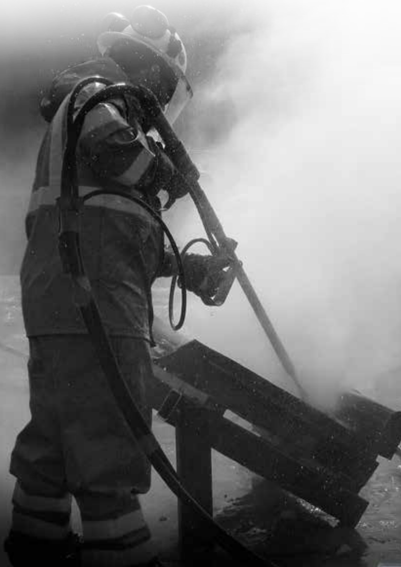
PAVEMENT MARKING REMOVAL
