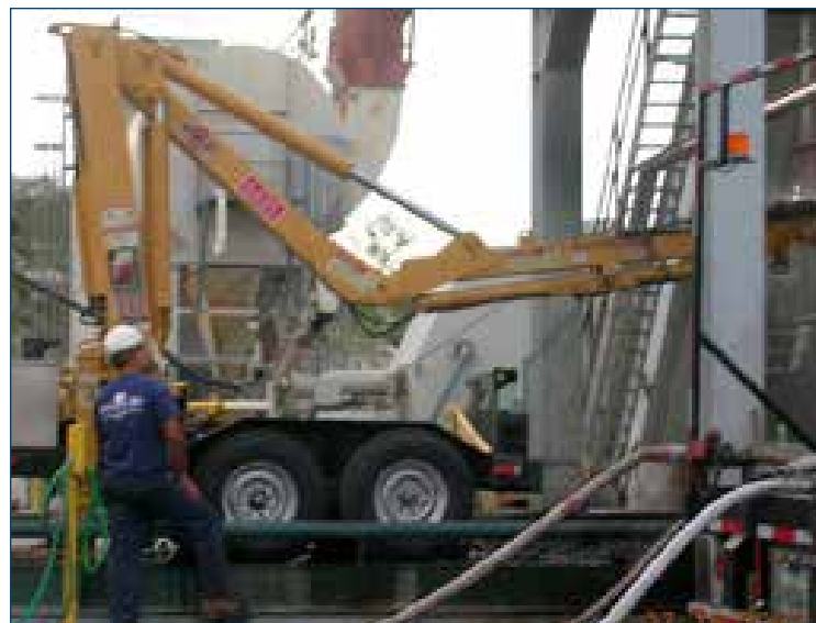
ASPHALT SILO CLEANING
